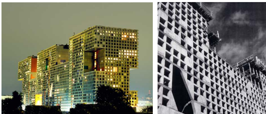
Figure 2. Simmons Hall undergraduate residence, MIT: View from Vassar Street, and exterior view of the “perfcon” structure during construction
